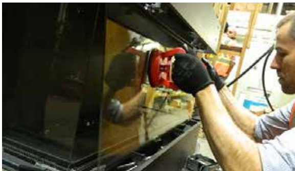
Handle front panel with supplied vacuum clamps
